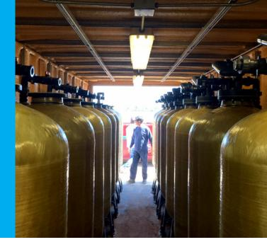
Purolite's SSTC60 operated in Al³+ form is a Shallow Shell™ technology resin featuring a solid core and functionalized outer shell specially designed for the selective removal of fluoride from water and waste water. The unique Shallow Shell design allows for effective removal of fluoride ions during the service cycle and efficient reversibility and clean-up of the resin during regeneration to give predictable and consistent performance and low leakage over time.
